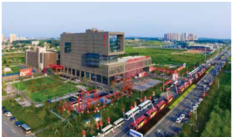
GiGo Holding head office building in Changchun City, Jilin Province, China
